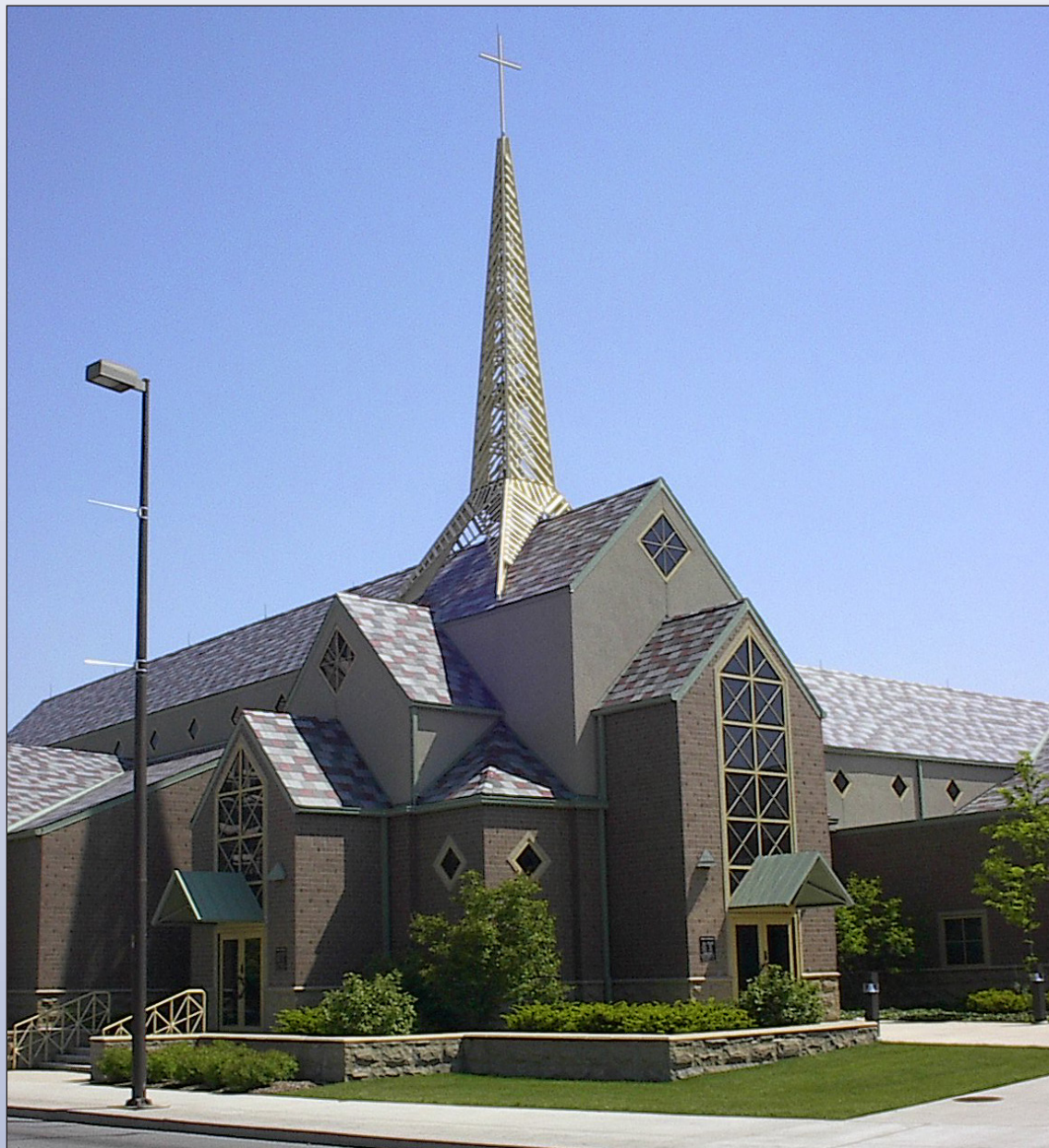
A cross-section of Catholics from all over the city of Fort Wayne considers St. Mary Mother of God Church, downtown, their home parish.
