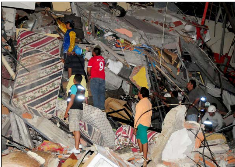
CNS photo/Paul Ochoa, Reuters People search for victims in the rubble of a destroyed building in Manta, Ecuador, April 16 after an 7.8-magnitude earthquake struck the region. At least 400 people died, nearly were 3,000 injured and thousands were left homeless.
