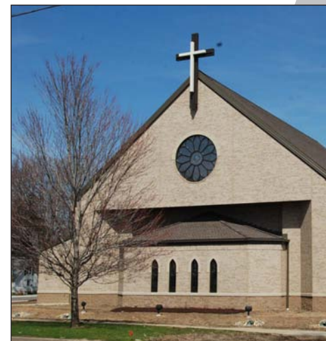
An external view of the new church.
