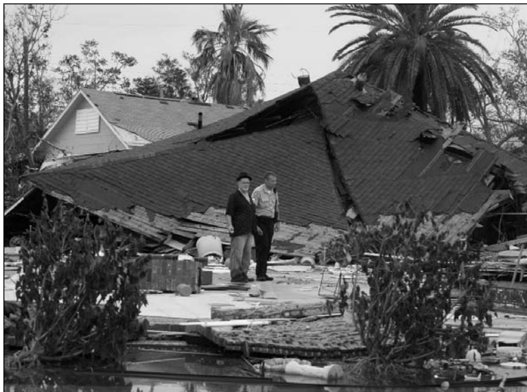
A police officer stands next to a resident as he surveys the damage caused by Hurricane Ike in Galveston, Texas Sept. 14. The hurricane hit the Texas and Louisiana coasts Sept. 13, causing extensive damage and flooding.
