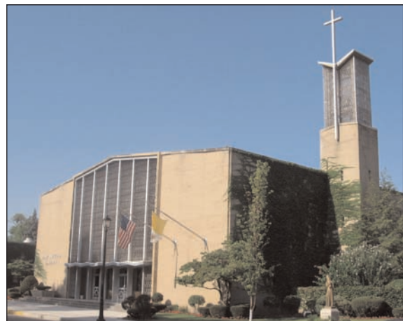
The St. Matthew Cathedral, the co-cathedral of the Diocese of Fort Wayne-South Bend, is located at 1701 Miami St. in South Bend.
