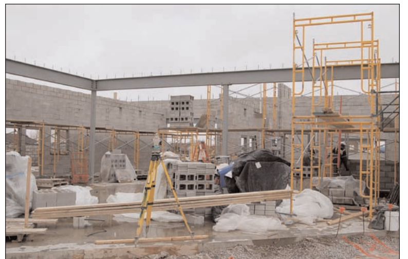
PROVIDED BY WEIGAND CONSTRUCTION
