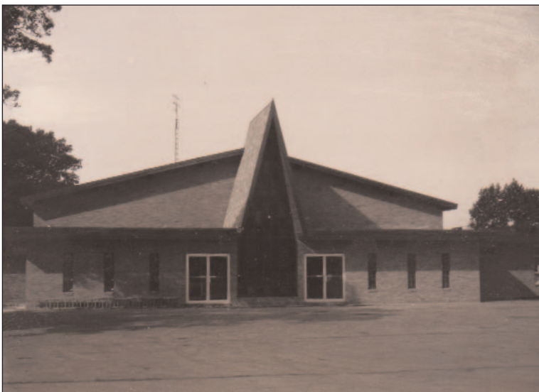
EXTERIOR OF ST. JOHN THE BAPTIST
