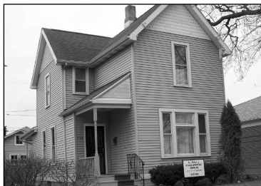
This house is now home to the parish food bank supported and staffed by St. Vincent de Paul volunteers. The food bank receives visitors every Thursday from 1-2 p.m. in a roomy and more homelike atmosphere.
