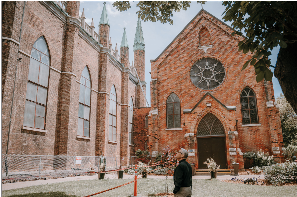
Father Maurice Restivo stands near Our Lady of the Assumption Church in Windsor, Ontario, June 14. Founded in 1767, the Canadian church needs $20 million in repairs.
