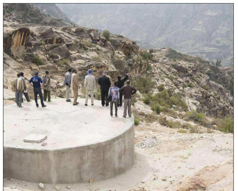
The group visits a large CRS water catchment project site in Salam Genet, Ethiopia, March 6. The site uses terraces to trap runoff rainwater and channel into a large cistern, pictured here. The water flows to taps just below this cistern and can be used for both agriculture and drinking, serving 400 families in this arid region of Tigray.
